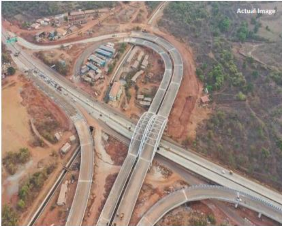
Trumpet Interchange Construction WIP
