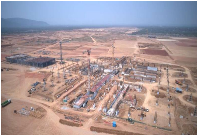
Passenger Terminal Building
